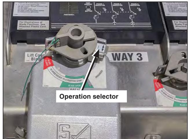
Figure 14. The operation selector In the far right position.
