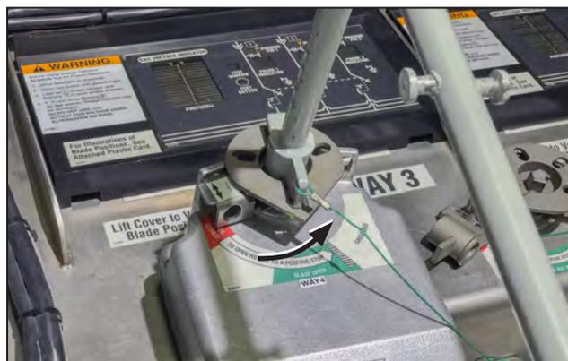
Figure 21. Grounding the load-interrupter switch (or fault interrupter).
