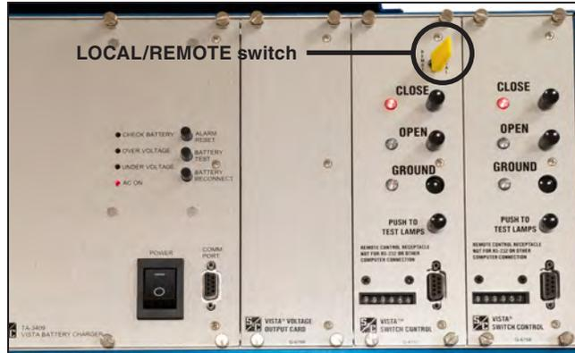
Figure 26. The motor operator control rack.
