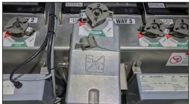
Figure 33. In the far left position, the operation selector allows operation between Open and Grounded positions.
