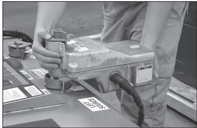
Figure 36. Lift the motor operator.
