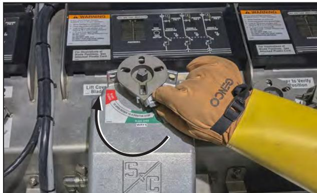
Figure 20. Rotating the operation selector to far left enables operation to Grounded position.
