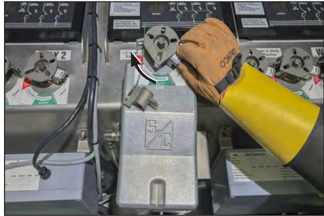
Figure 31. Rotate the operation selector out of the way.
