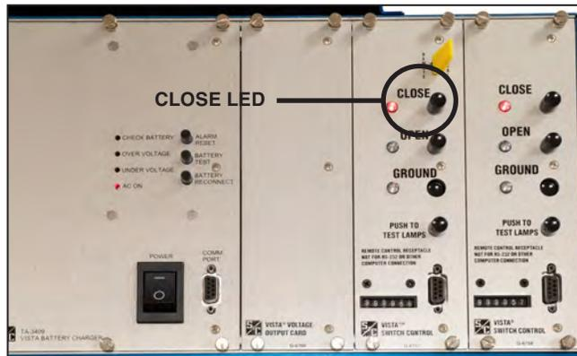
Figure 28. The Close position indicator on the motor control board matches the motor operator position.
