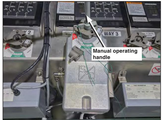
Figure 29. Remove the operating handle.
