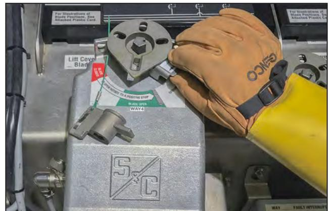
Figure 15. Rotate the operation selector out of the way.
