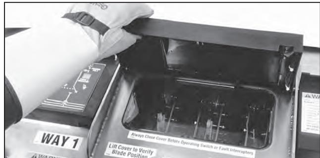
Figure 12. The window cover lifts for viewing of switch or fault-interrupter blade positions.
