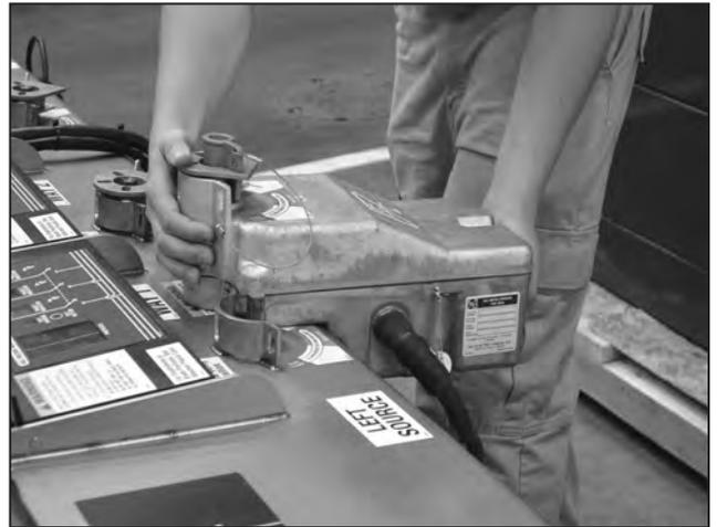
Figure 38. Reposition the motor operator.
