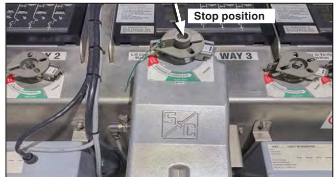
Figure 30. Replace the electrical-operation mechanical blocking key.
