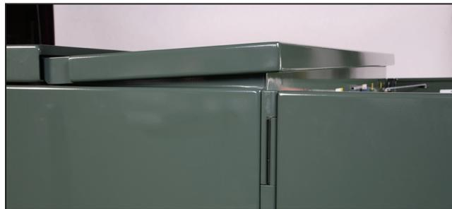
Figure 4. Roof section disengaged from pad-mounted gear enclosure.
