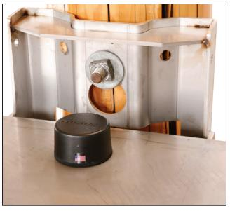
Figure 16. GPS antenna installed on the top of the IntelliRupter fault interrupter base.
