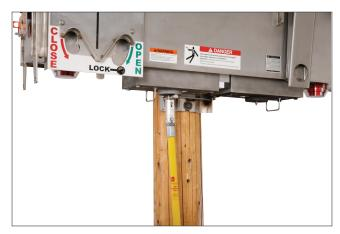
Figure 1. Inserting the handling fitting into the module latch.
