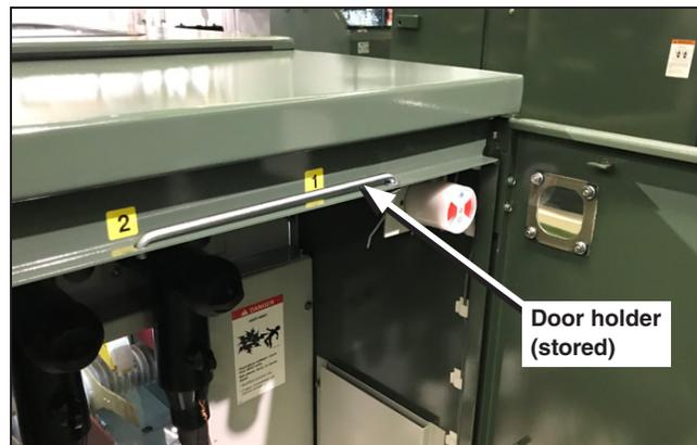
**Figure 7.** The door holder placed in the storage position to allow the door to close.
