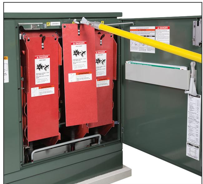
Figure 19. Removing or replacing the dual-purpose front barrier with the Grappler tool.
