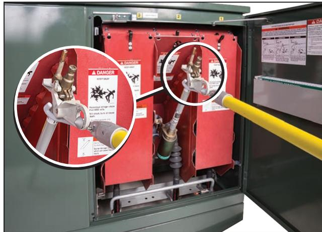
**Figure 21.** Installing a fuse using a Grappler Handling Tool. The inset image shows a close-up of a Grappler tool in position to install the fuse.
