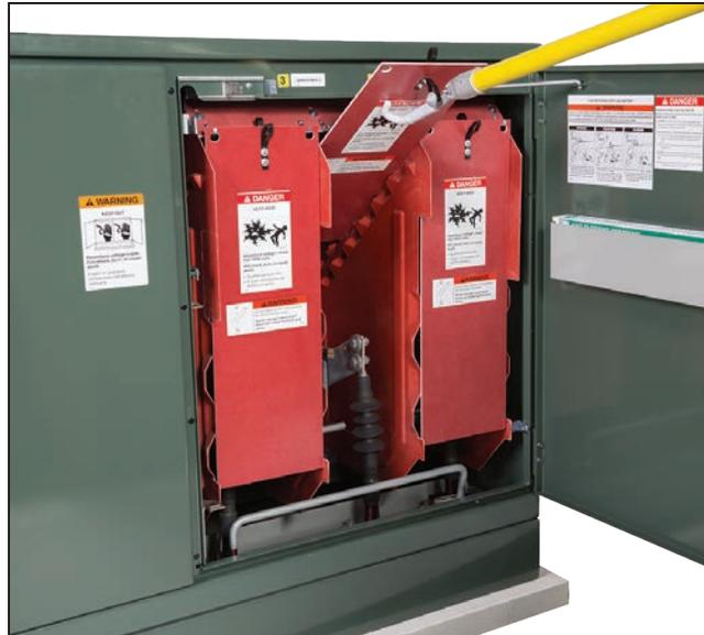
**Figure 20.** Inserting the dual-purpose front barrier into the “Slide-in” position using a Grappler tool.
