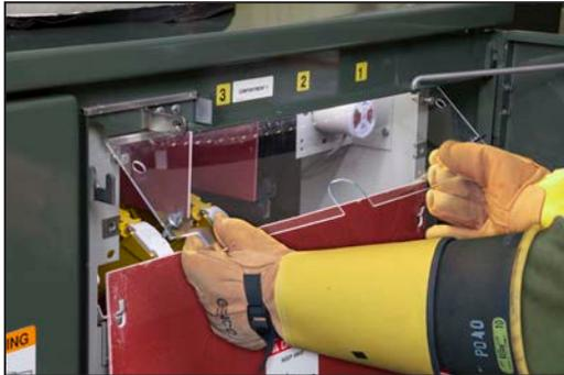
**Left-hand door retainer**—Rotate the latch upward to open the door. To secure the left-hand door closed, rotate the latch downward over the stop mounted on outer edge of the door.
