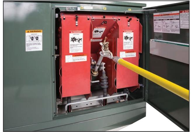
Figure 22. A fuse installed in mounting in the Open position.
