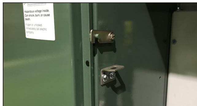
**Figure 8.** The left-door latching mechanism engaged.
