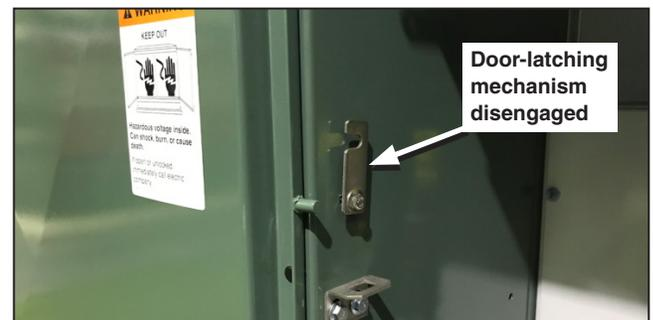
**Figure 4.** The left-door latching mechanism disengaged.
