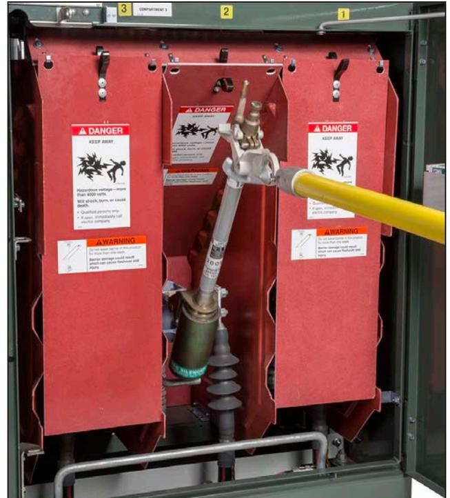
**Figure 29.** Removing a fuse from its hinge with a forward and upward lifting motion.
