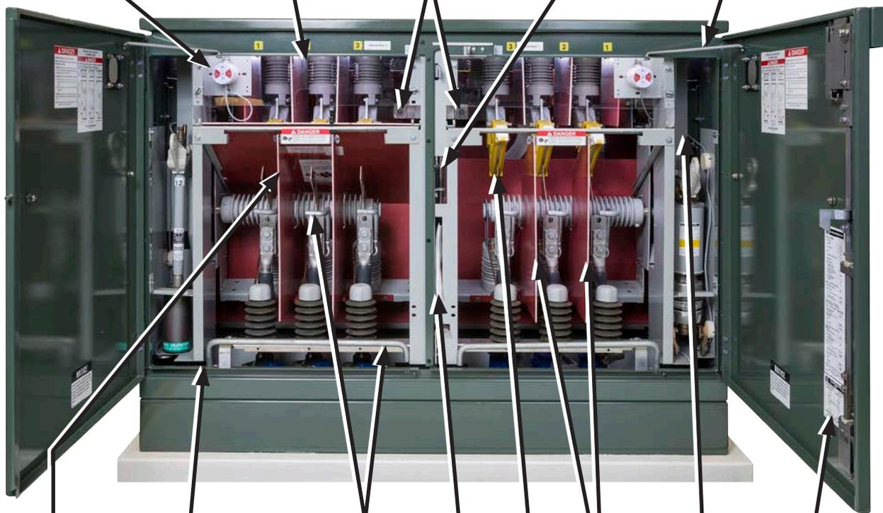
**Ground pad** on the inside at the bottom the door stile in each compartment accommodates connectors for attachment of cable concentric-neutral ground leads and ground studs.
