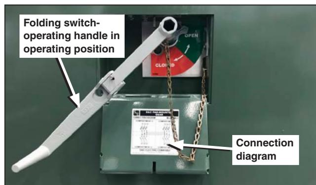
Figure 12. The switch operating handle installed.
