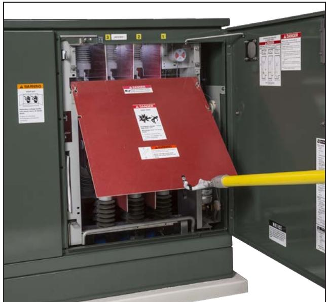
Figure 15. A Grappler Handling Tool being used to lift the barrier. Note the door holder is in place and the adjacent door is latched closed to reduce exposure to high voltage.
