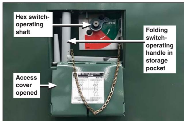
Figure 11. The access cover door is open.
