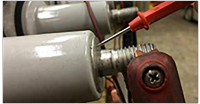
**Figure 61. Take the measurement from the flat current-carrying surface of the bushing.●**
