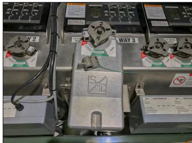
Figure 33. In the far left position, the operation selector allows operation between the Open and Grounded positions.
