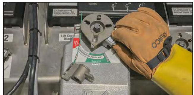
Figure 15. Rotate operation selector out of the way.
