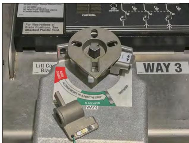
Figure 19. Motor operator recharged and in the Open position.
