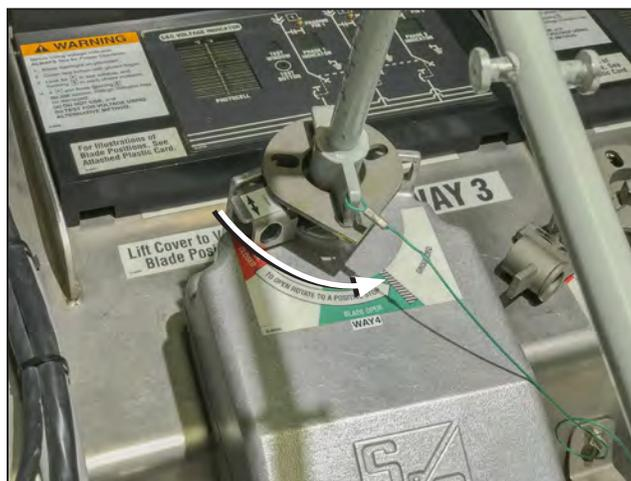
Figure 21. Ground the load-interrupter switch (or fault interrupter).
