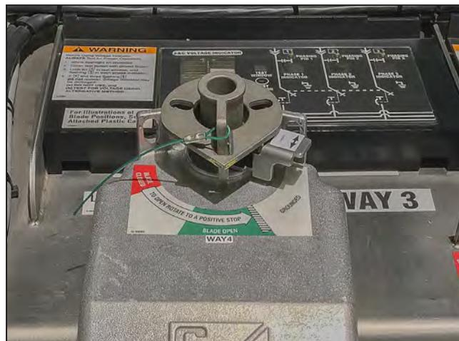
Figure 28. Switch in Open position.
