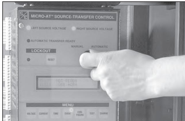
Figure 27. MANUAL/AUTOMATIC switch on Micro-AT control.
