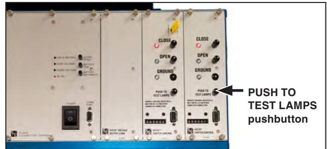
Figure 34. The PUSH TO TEST LAMPS pushbutton.
