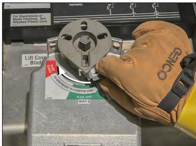
Figure 20. Rotating the operation selector to far left enables operation to Grounded position.
