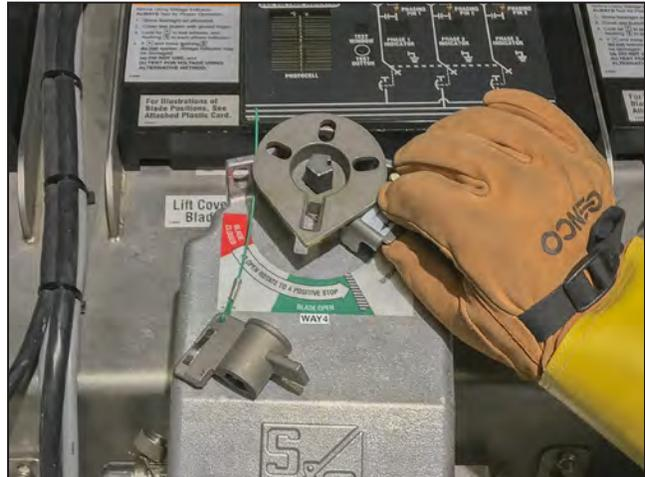
Figure 31. Rotate the operation selector out of the way.
