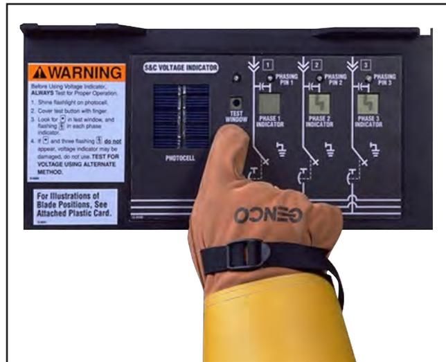
Figure 49. If one or more PHASE indicators does not show a flashing lightning bolt during testing, the VOLTAGE indicator may be damaged. Test for voltage using an alternate method.
