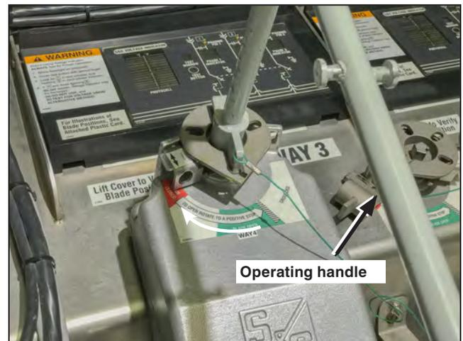
Figure 29. Remove the operating handle.
