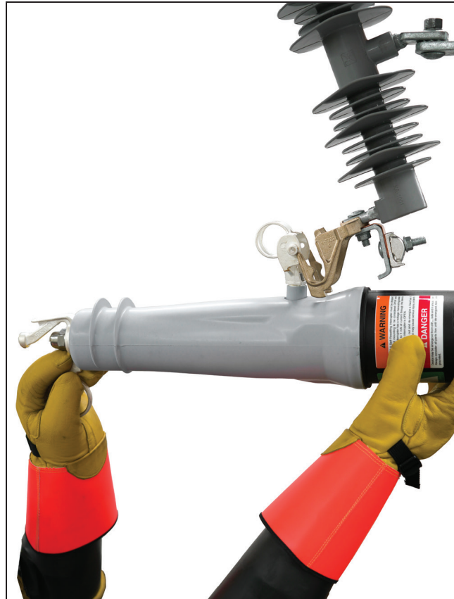
Figure 14. Removing the VacuFuse II interrupter with gloved hands.
