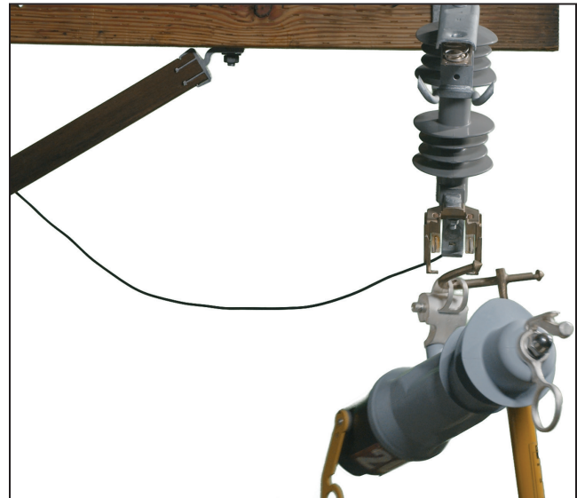
Figure 9. Using a Talon tool during installation.
