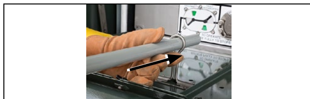
Figure 14. Insert the handle through the guide ring and attach it to the shaft of the operating mechanism.
