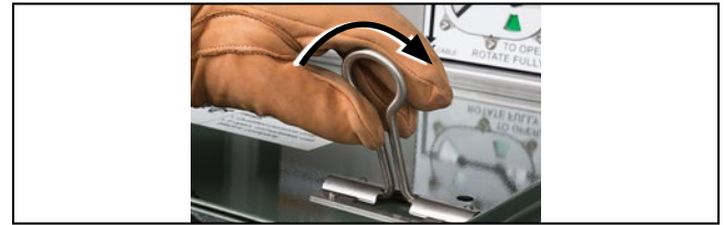
Figure 19. Rotate the operating handle guide ring to the active (up) position (a); insert the handle through the guide ring and attach it to the shaft of the operating mechanism.
