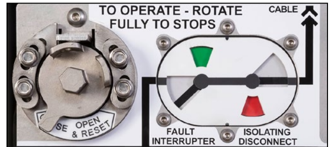
Figure 18. The POSITION indicator after a fault has occurred. The fault interrupter is open, and the isolating disconnect is closed.
