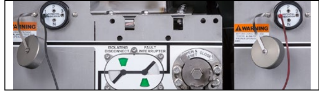
Figure 31. Measure the phase-to-phase voltage between Test Jacks 1, 2 and 3 of the first way and Test Jack 1 of the second way.
