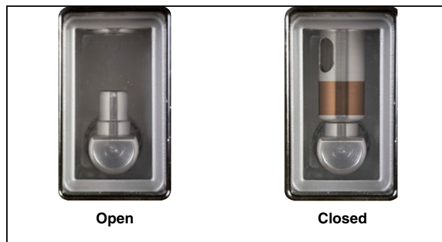
Figure 17. The visible-open gap (isolating disconnect) is easy to see through large viewing windows.
