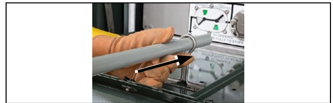
Figure 20. Rotate the operating handle guide ring to the active (up) position (a); insert the handle through the guide ring and attach it to the shaft of the operating mechanism.
