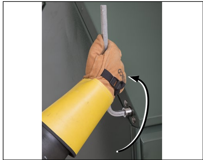
Figure 8. Using a pentahead socket wrench or tool, rotate the bolt latching mechanism 360° counterclockwise to unlock the hinged roof.
