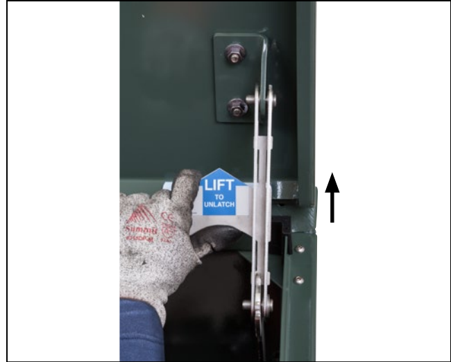
Figure 36. While pushing up on the hinged roof, release the latch on the “hold-open” mechanism.
