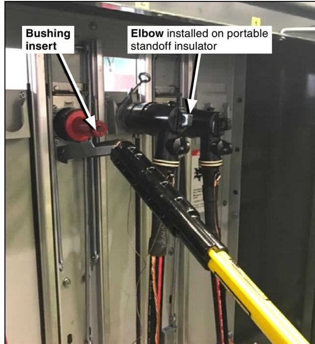
Figure 10. Raising the mechanical interlock to unlock the TransFuser Mounting.
