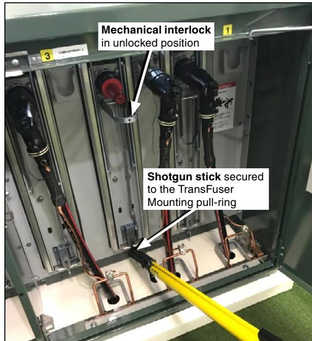
Figure 11. Unlatching (or latching) the TransFuser Mounting in the Closed position.
