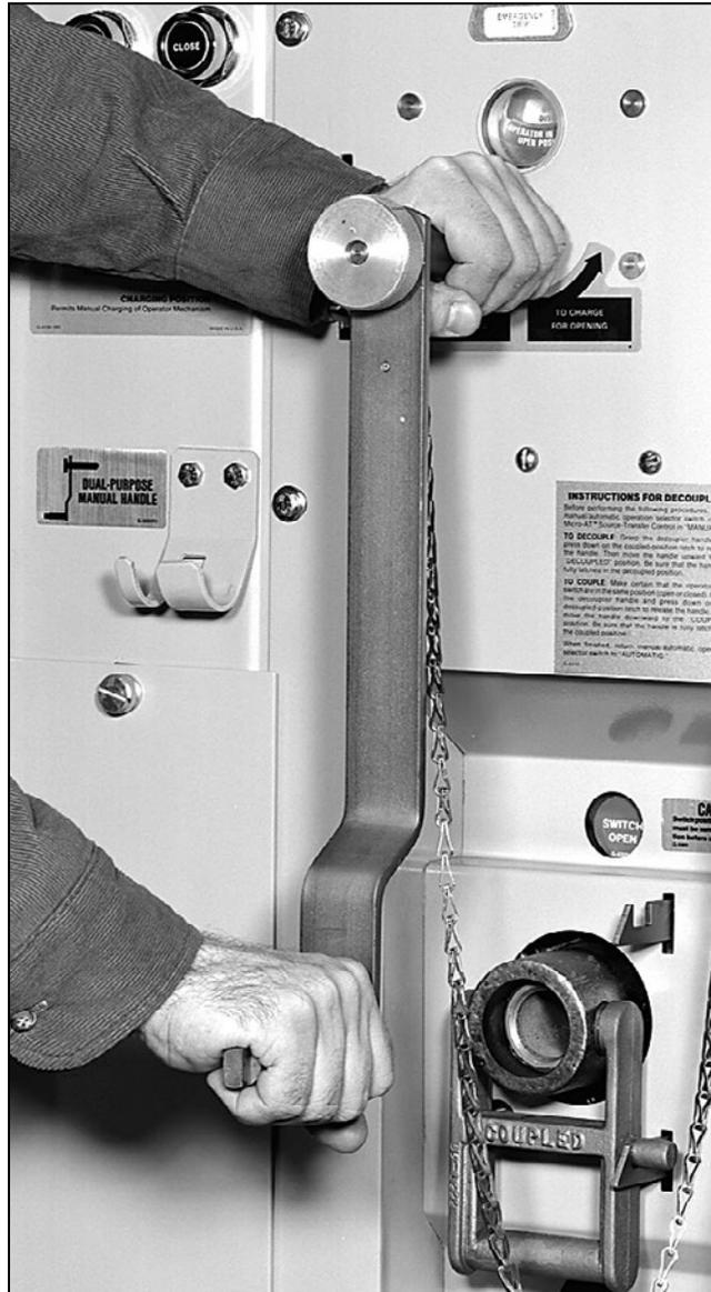
Figure 7. Dual-purpose manual handle on the charging shaft.
