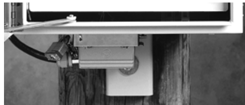
Figure 4. FIC plug on the bottom of the enclosure.
