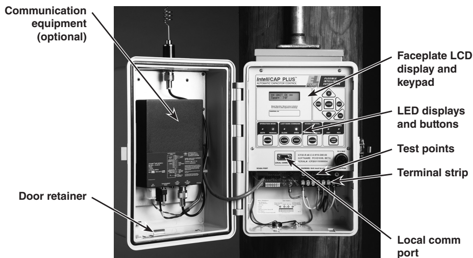
Figure 2. IntelliCap Plus Control with the door open.
