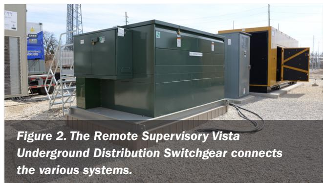
**Figure 2. The Remote Supervisory Vista Underground Distribution Switchgear connects the various systems.**
