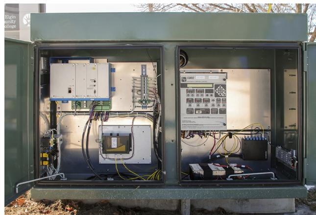
**View of automation equipment inside S&C Vista switchgear.**
