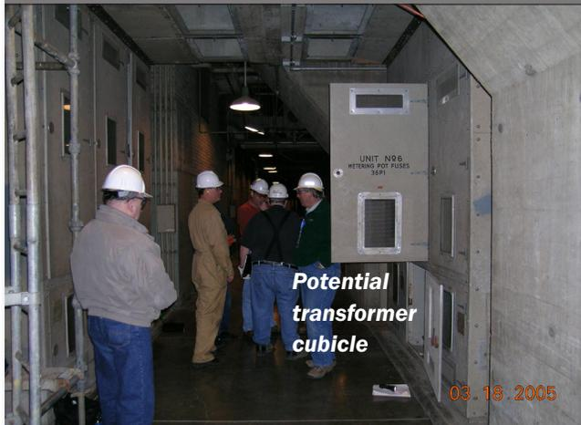
*S&C Type RR Potential Transformer Protective Combination installed in potential transformer cubicle. The potential transformer (not visible) is located at the bottom of the cubicle. The S&C Type DLC Liquid Power Fuse has been removed from the mounting in this photo.*
