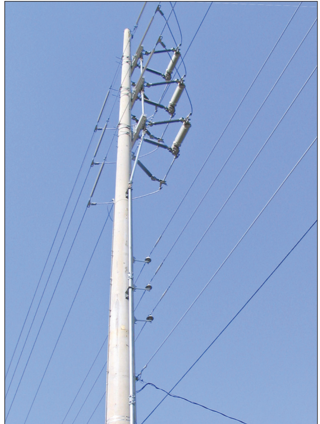
A 115-kV Line-Rupter Switch specially modified by S&C's Technical Services for installation "phase over phase" in a transmission line sectionalizing application. Furnished with silicone insulators to reduce weight.
