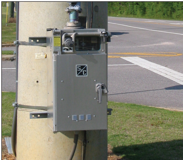
A Type LS-2 Switch Operator for use with the Line-Rupter Switch.
