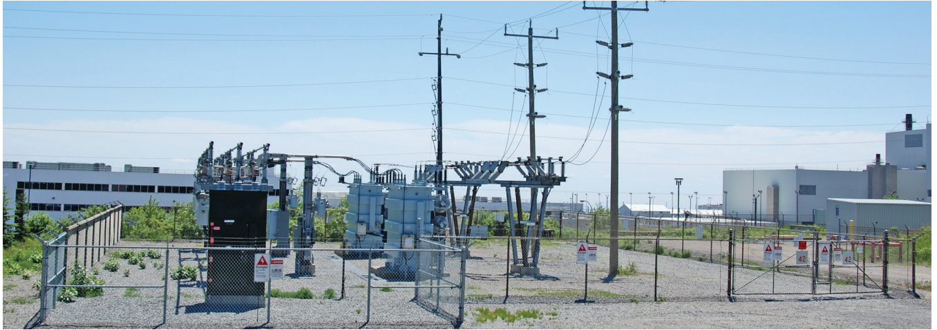
Figure 2. An open-air substation. Footprint: 50 feet \times 50 feet (15 m \times 15 m). Requires a safety fence and ground grid.
