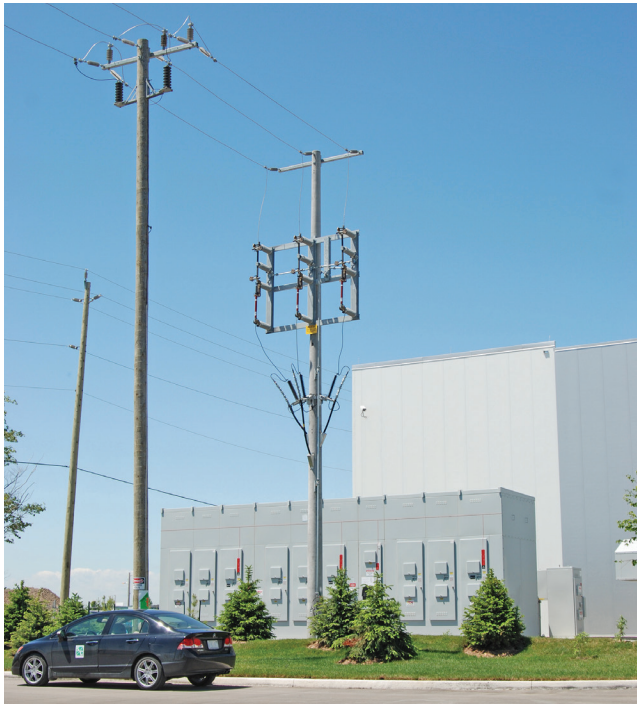
Figure 3. A three-bay S&C Custom Metal-Enclosed Switchgear lineup. Footprint: 28 feet \times 22 feet (8.5 m \times 6.7 m). No safety fence or ground grid needed.
