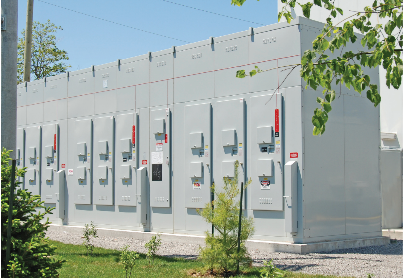
Figure 1. A typical 46-kV S&C Custom Metal-Enclosed Switchgear lineup.
