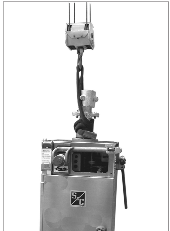
Figure 1. Lifting the switch operator.
