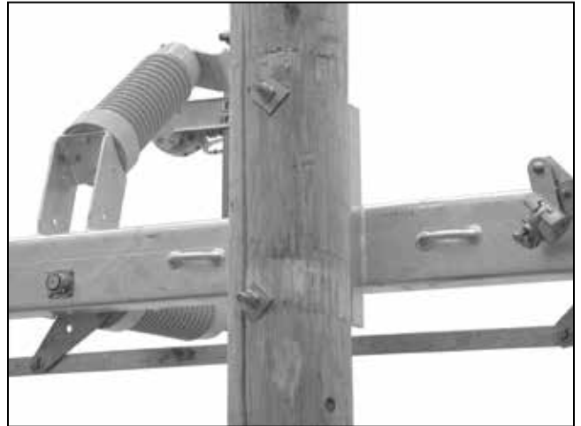
Figure 9. Bolting the switch.
