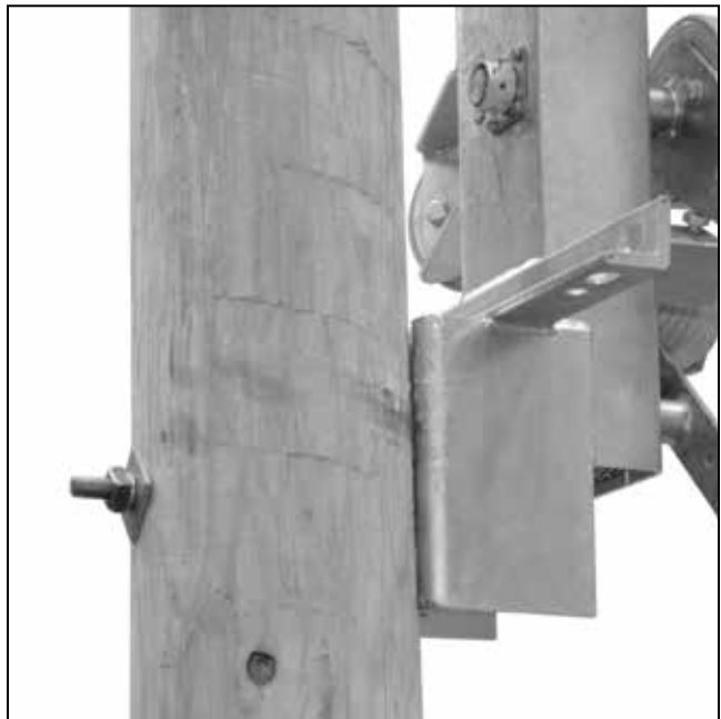
Figure 16. Bolting the switch.
