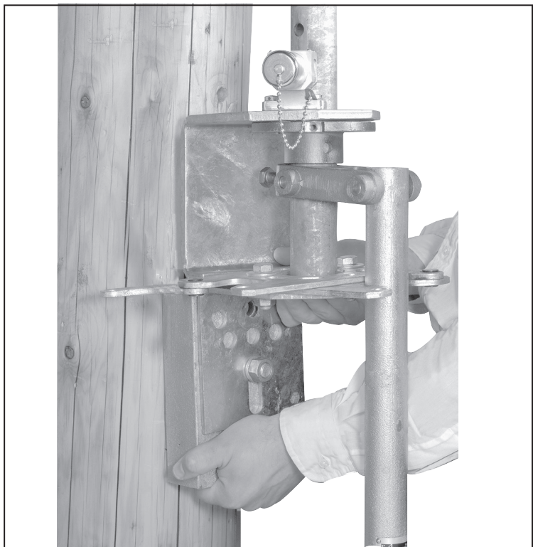
Figure 29. Position the interlock bracket, locking disc, operating-handle assembly, and foot-bearing assembly onto the lowest vertical operating-pipe section.
