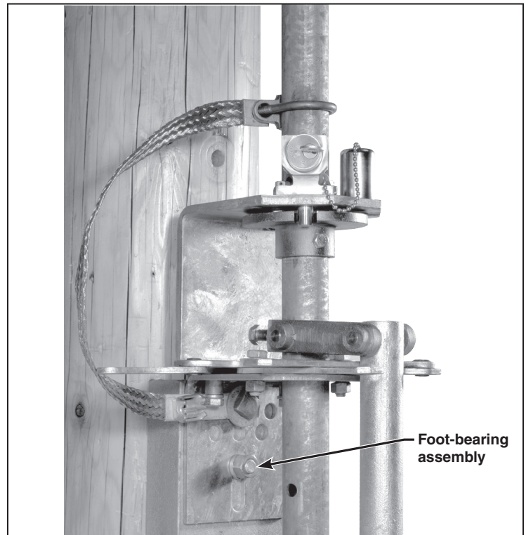
Figure 30. Attach the foot-bearing assembly.
