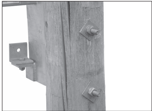
Figure 21. Bolting the switch.
