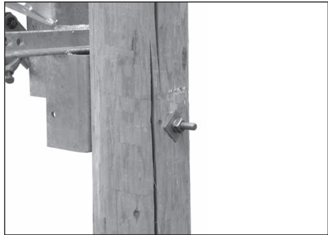
Figure 16. Bolting the switch.
