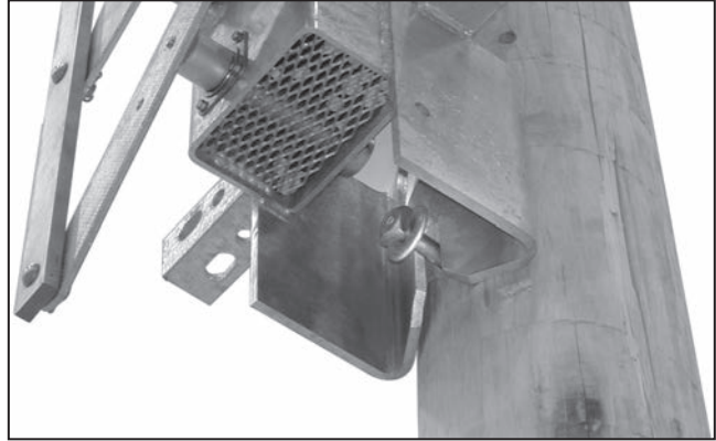
Figure 15. Guiding the switch.
