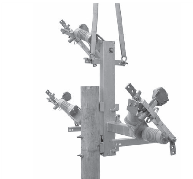
Figure 19. Hoisting the switch into position.
