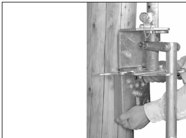
Figure 23. Position the interlock bracket, locking disc, operating handle assembly, and foot-bearing assembly onto the lowest vertical operating-pipe section
