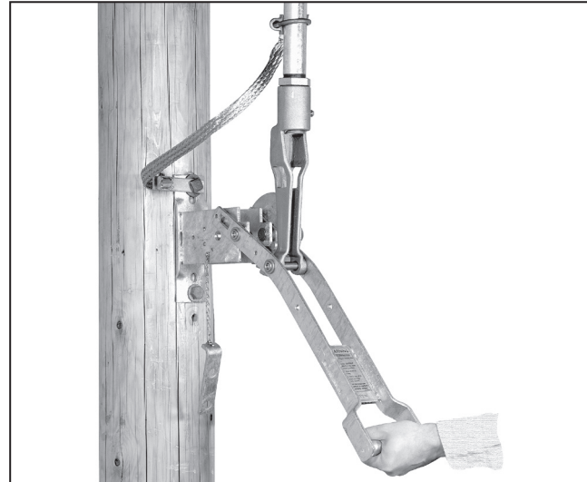
Figure 20. Verifying the stack has been taken up in the operating linkage.
