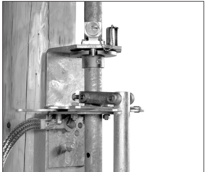
Figure 13. Attach the foot-bearing assembly.
