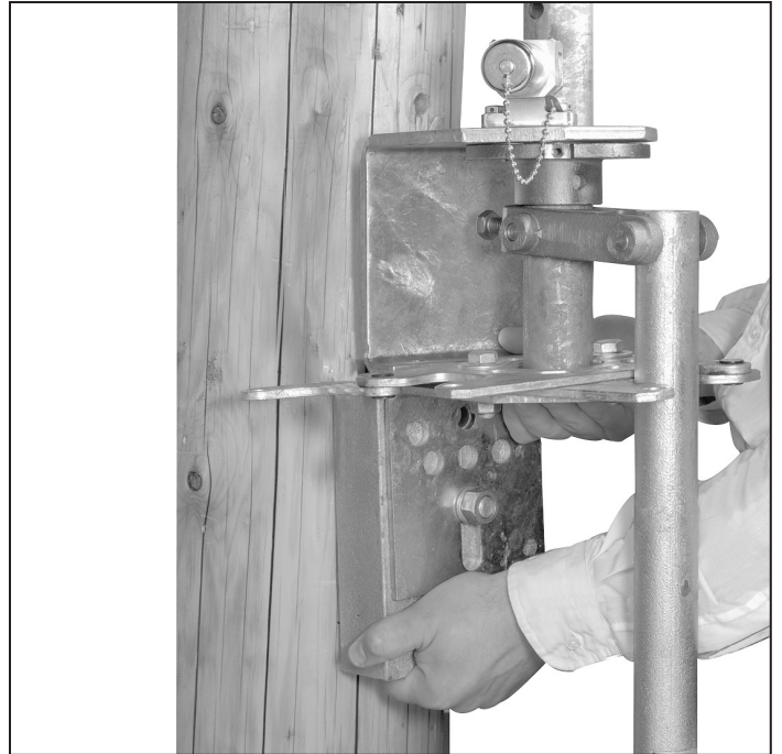
Figure 12. Position the interlock bracket, locking disc, operating-handle assembly, and foot-bearing assembly onto the lowest vertical operating pipe section.
