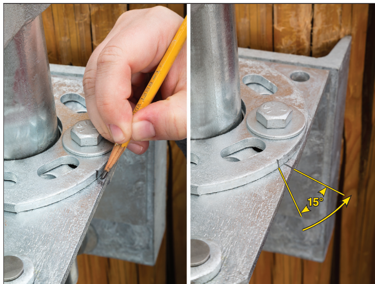
Figure 22. Mark the stop plate, then loosen the hardware and rotate the closed stop plate backward approximately 15 degrees.
