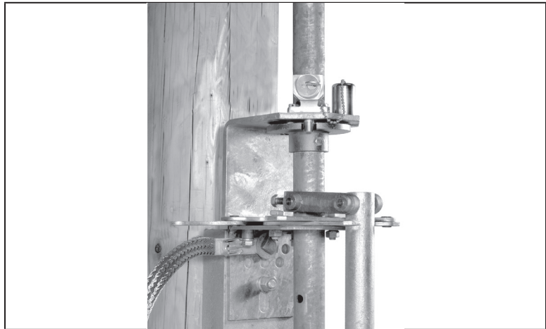
Figure 16. Attach the foot-bearing assembly.
