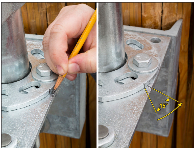
Figure 29. Mark the stop plate, and then loosen the hardware and rotate the closed stop plate backward approximately 15 degrees.
