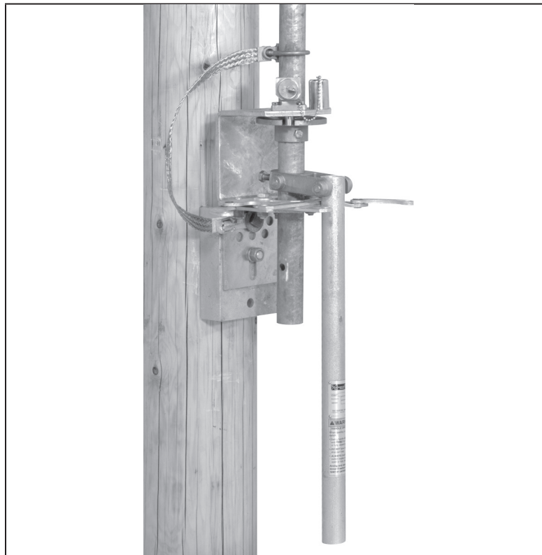
Figure 46. Disengage the key interlock bolt.
