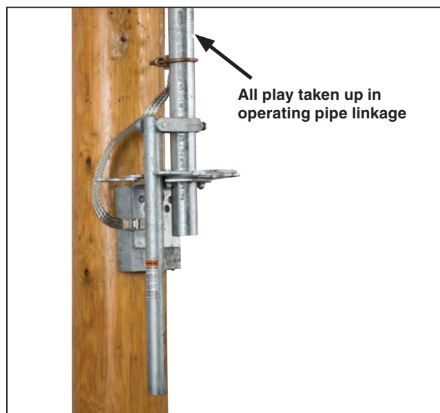
Figure 44. Verify the handle fits into the open stop plate.
