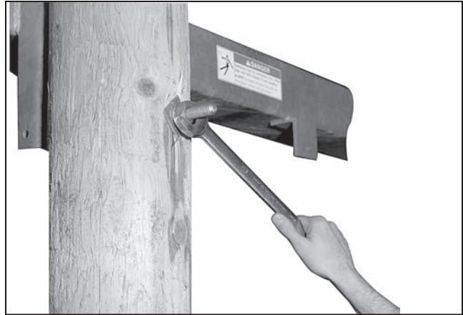
Figure 18. Tighten the bolts.
