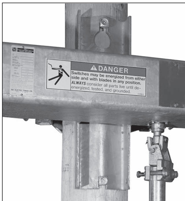
Figure 27. Attach the universal coupling to the switch drive shaft.
