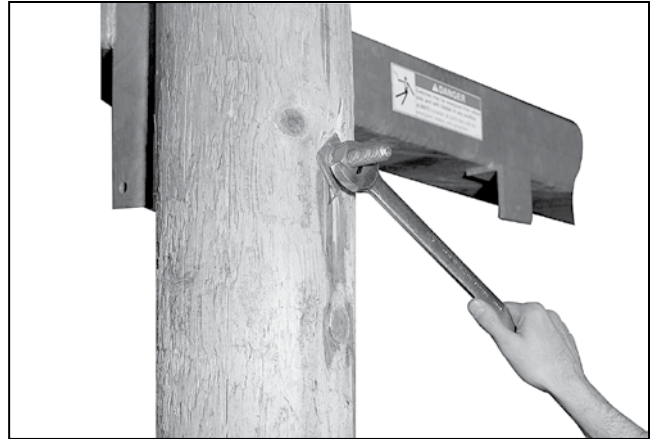
Figure 18. Tighten the bolts.
