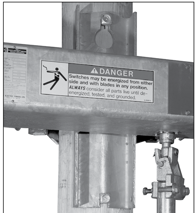
Figure 27. Install the uppermost section of the vertical operating pipe.
