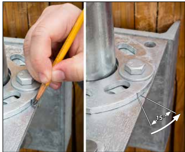
Figure 43. Torque bolts securing the stop plates to the support plate.
