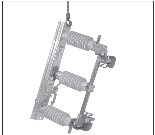
Figure 6. Hoisting the switch pole into position.
