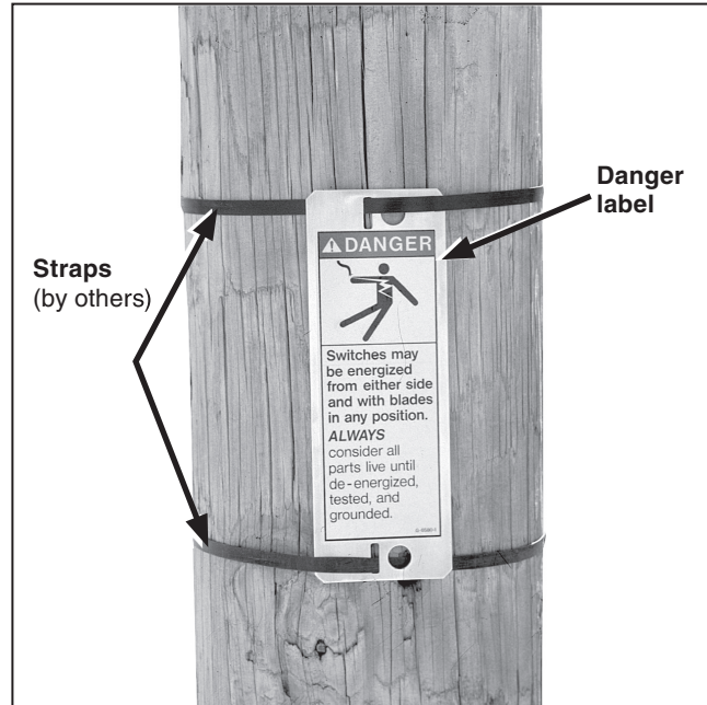
Figure 38. Attaching the danger label to the pole or structure.
