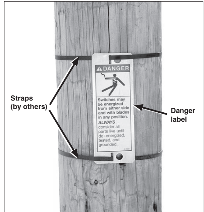
Figure 42. Attaching the danger label to the pole or structure.
