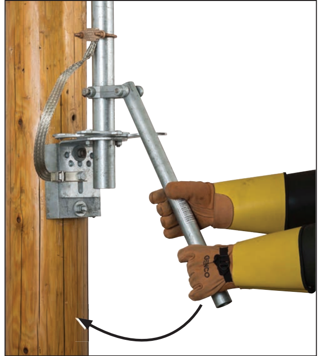
Figure 32. Move the handle between open and closed stop plates. The handle should fit tightly in the closed plate.
