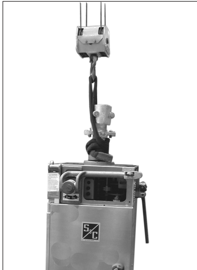
Figure 1. Lifting the switch operator.
