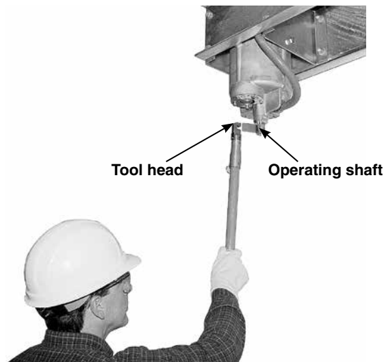
Figure 51. Guide the hooked end of the charging tool between the ears of the operating shaft.
