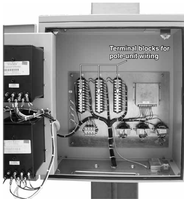
Figure 19. Connect pole-unit wiring to terminal blocks in control cabinet, in accordance with the wiring diagram furnished.
