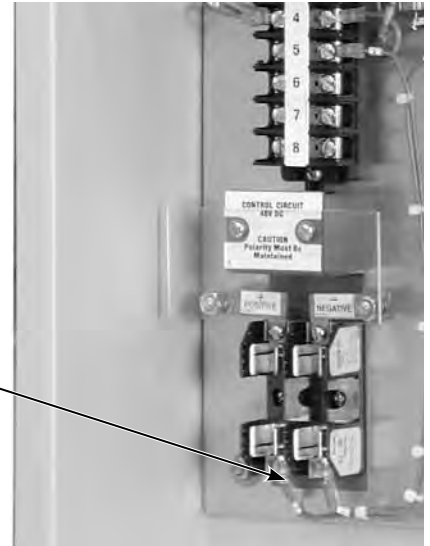
Figure 74. Connect the control-power wiring to the terminal blocks in the enclosure.
