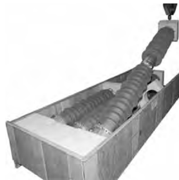
Figure 31. Pull the pole-unit carefully upward.
