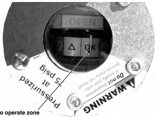
Figure 5. Check that the gas-pressure gauge on each pole-unit is in the “OK” to operate zone.
