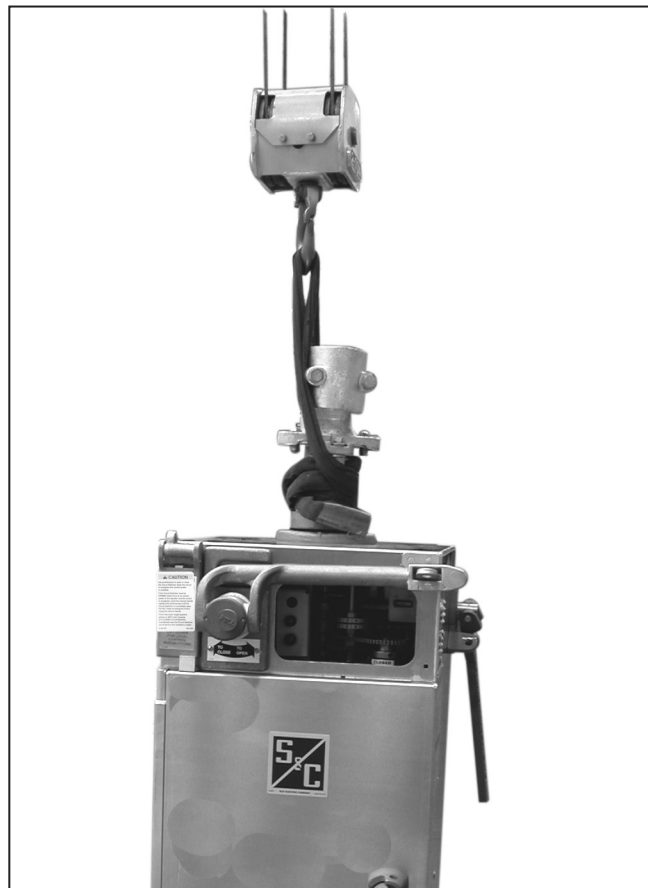
Figure 1. Lifting the switch operator.
