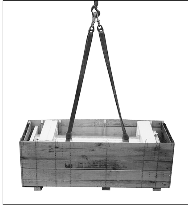
Figure 7. Removing the replacement interrupter from the from shipping crate.
