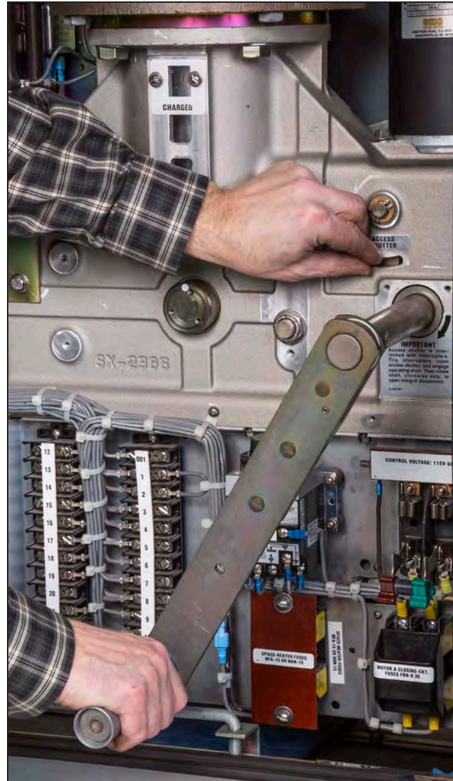
Figure 31. Using the manual charging handle to recharge the opening and closing springs and the open disconnect.
