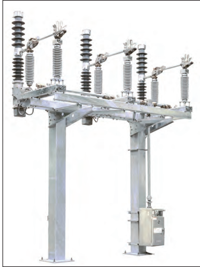
Figure 83. Completed Mark VI Circuit-Switcher installation.
