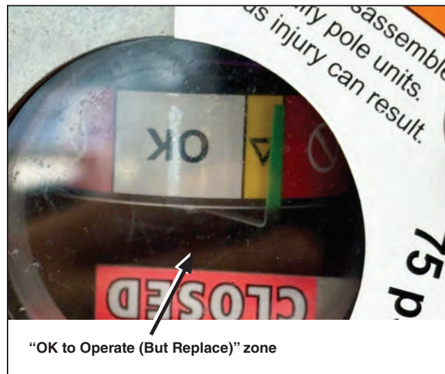
Figure 87. Gauge needle in yellow OK to Operate (but Replace) zone.
