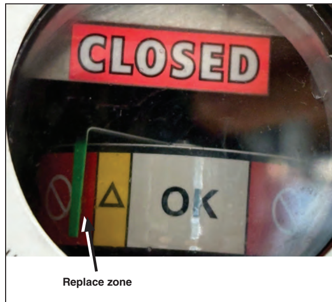
Figure 75. Gauge needle in red Replace zone.
