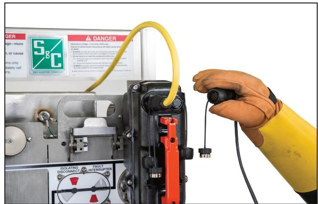
Figure 3. Attaching the Vista SD switchgear portable motor control pendant cable to motor operator.
