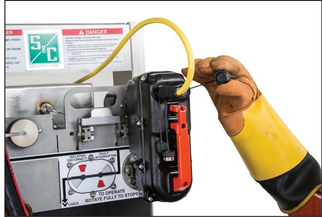
Figure 2. Removing the submersible cap.
