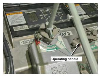
Figure 29. Remove the operating handle.
