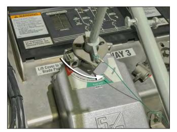
Figure 21. Ground the load-interrupter switch (or fault interrupter).
