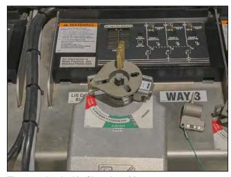
Figure 23. Locked in Closed position.
