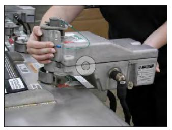
Figure 39. Lift the motor operator.
