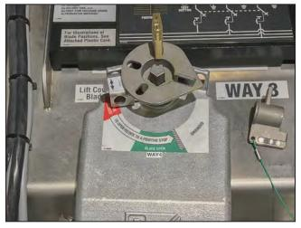
Figure 25. Locked in Grounded position.
