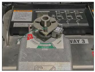
Figure 28. Switch in Open position.
