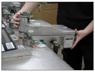
Figure 41. Reposition the motor operator.
