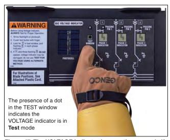
Figure 47. The VOLTAGE indicator is operating properly if a dot appears in the TEST window and a flashing lightning bolt appears in each PHASE indicator.
