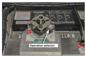
Figure 14. Operation selector in the far right position.
