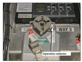
Figure 32. In the far right position, the operation selector allows operation between the Closed and Open positions.
