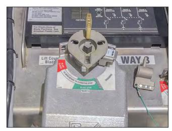
Figure 24. Locked in Open position.
