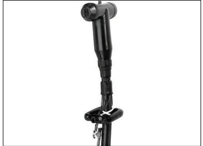
Figure 83. Current sensors placed around cable's grounded concentric neutral.●
