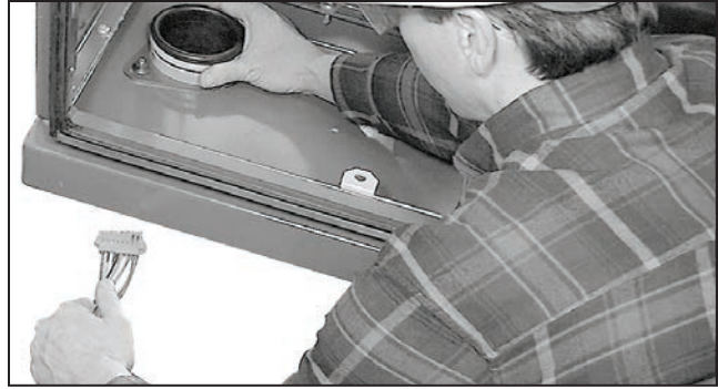
Figure 58. Channel cables through wire pass.
