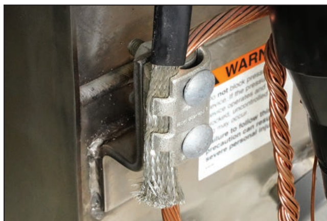
Figure 113. Connect shielded cable to tank ground.
