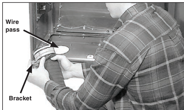
Figure 119. Place the holding brackets in the grooved channel of the conduit.
