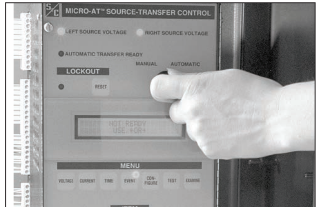
Figure 38. The MANUAL/AUTOMATIC switch on the Micro-AT Source-Transfer Control.
