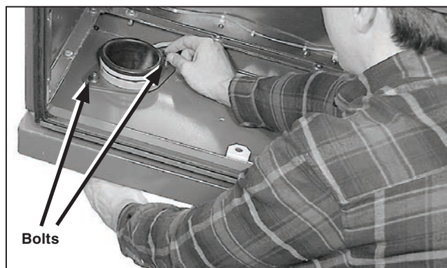
Figure 120. Install and secure the assembly through the wire pass.
