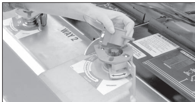
Figure 67. Insert the mechanical blocking key.
