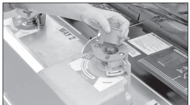
Figure 98. Insert the mechanical blocking key.
