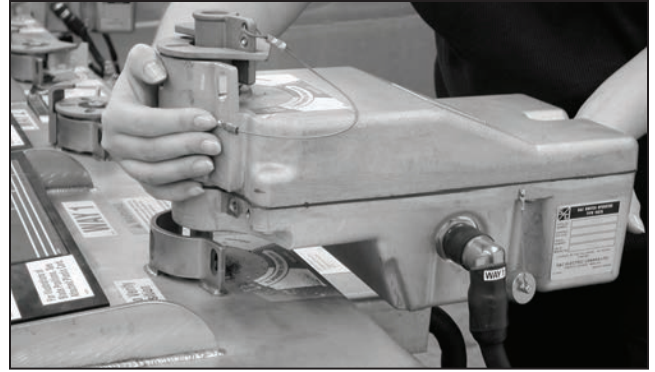
Figure 95. Place the motor operator over the operating shaft on the gear.
