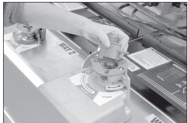
Figure 39. Remove the mechanical blocking key.
