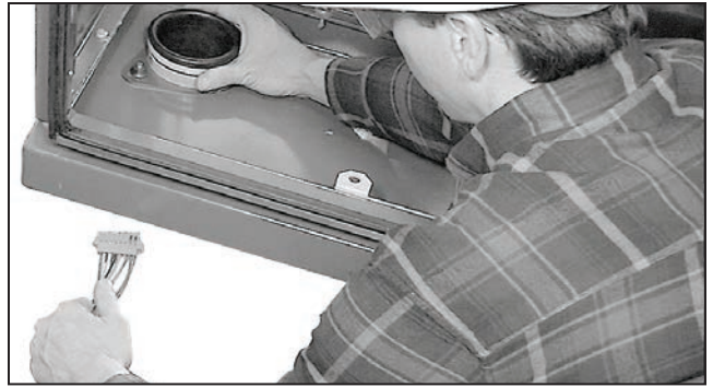
Figure 121. Channel the cables through the wire pass.
