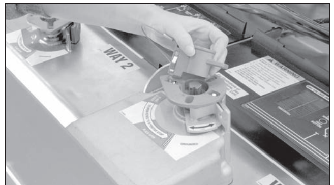
Figure 130. Insert the mechanical blocking key.
