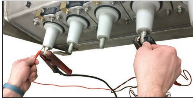
Figure 139. Connecting the resistance measuring device.●
