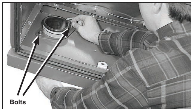
Figure 57. Install and secure the assembly through the wire pass.
