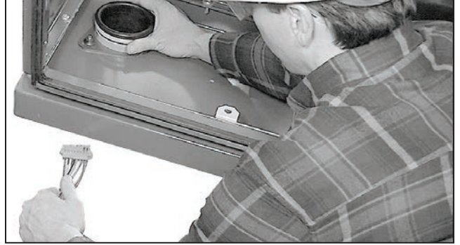
Figure 89. Channel the cables through the wire pass.
