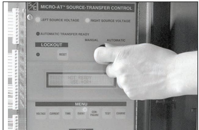
Figure 135. The MANUAL/AUTOMATIC switch on the Micro-AT Source-Transfer Control.
