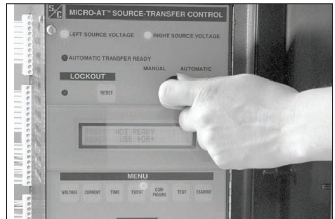
Figure 103. The MANUAL/AUTOMATIC switch on the Micro-AT Source-Transfer Control.
