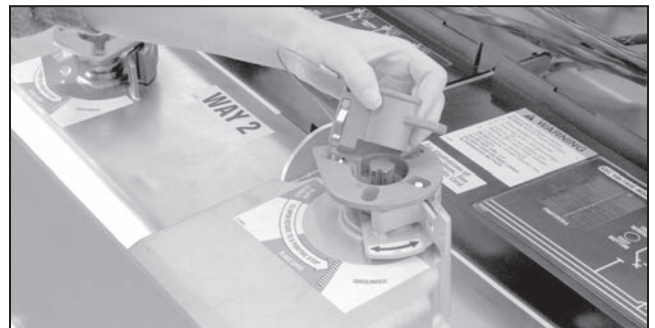
Figure 33. Insert the mechanical blocking key.
