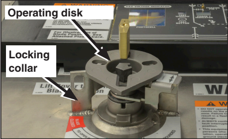
Figure 9. The operating disk locked to the back of the locking collar.
