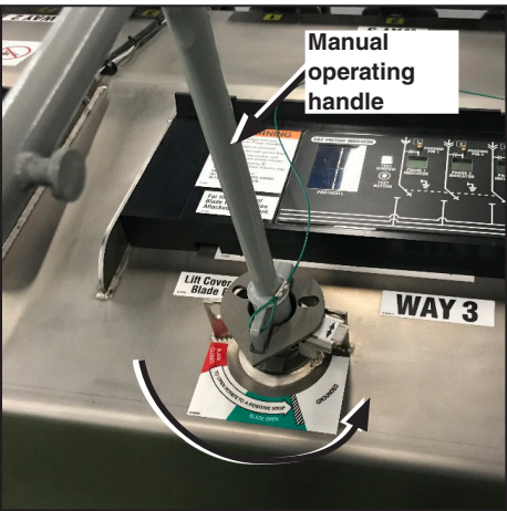
Figure 7. Opening the load-interrupter switch or fault interrupter.
