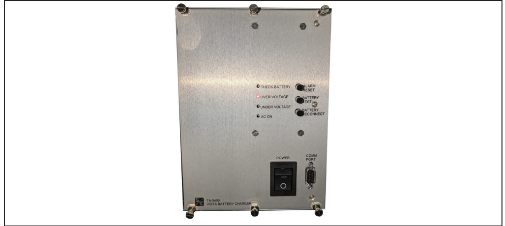
Figure 25. A battery charger with the OVER VOLTAGE indicator illuminated.
