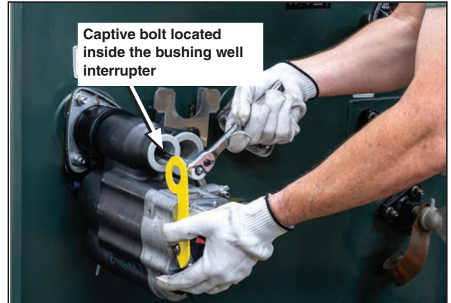
Figure 14. Loosen the captive bolt.
