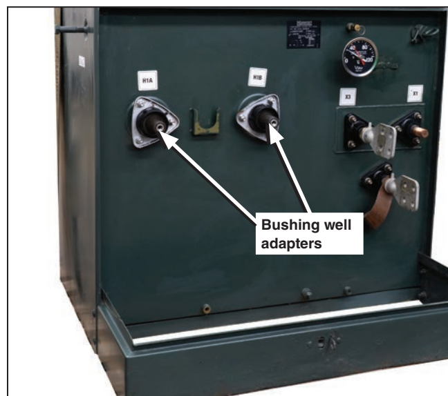
Figure 18. Remove the bushing well adapters.
