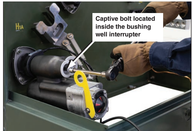
Figure 28. Loosen the captive bolt.
