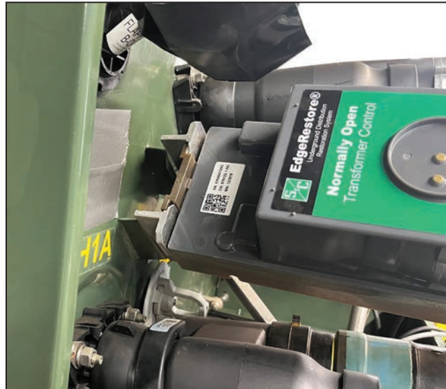
Figure 21. Remove the control from the parking stand.
