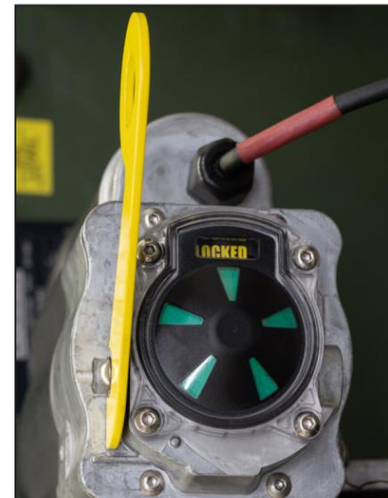
Figure 3. The bushing well interrupter in the Open and Locked position.
