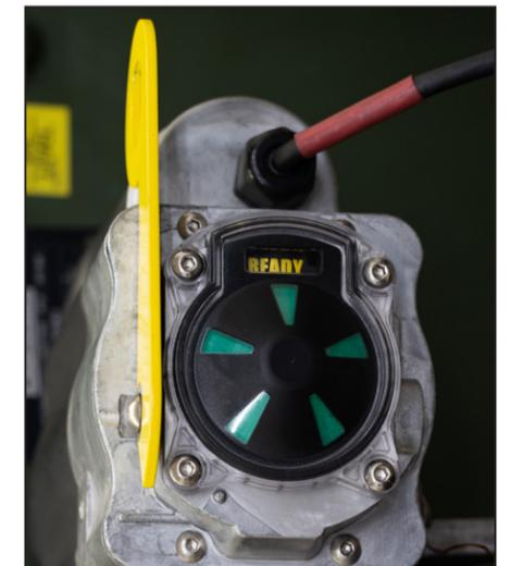
Figure 4. A bushing well interrupter in the Open and Ready position.
