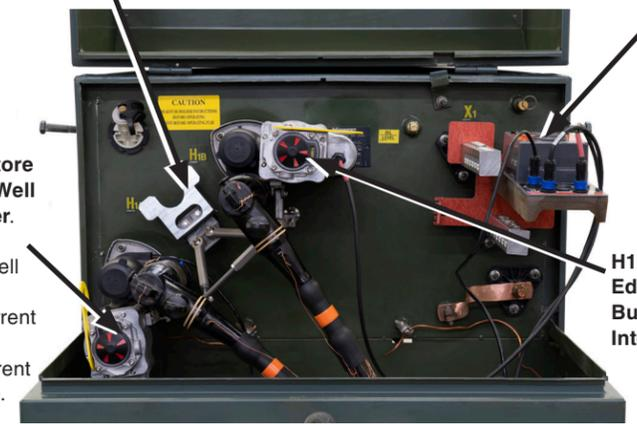
Figure 7. A complete EdgeRestore Underground Distribution Restoration System on an ANSI Type 2 transformer.
