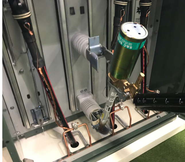
Figure 19. A fuse lowered into the cradle in preparation for latching to a TransFuser Mounting.
