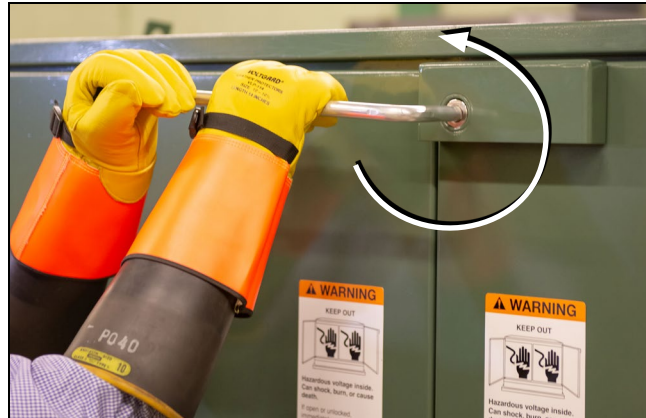
Figure 3. To unlock the doors, turn the pentahead socket wrench 60° counterclockwise against spring resistance until a “click” is heard and the wrench reaches its stop.
