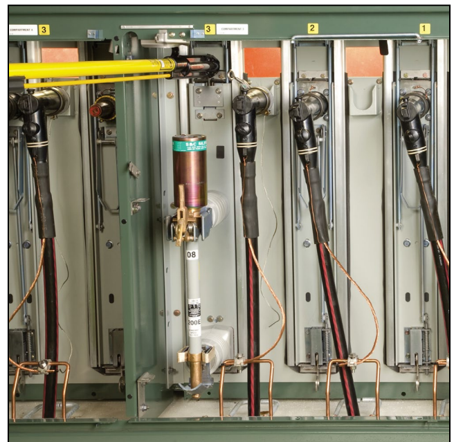
Figure 18. Latching (or unlatching) the TransFuser Mounting in the Open position.
