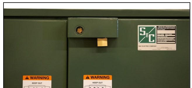
Figure 9. The enclosure doors padlocked.
