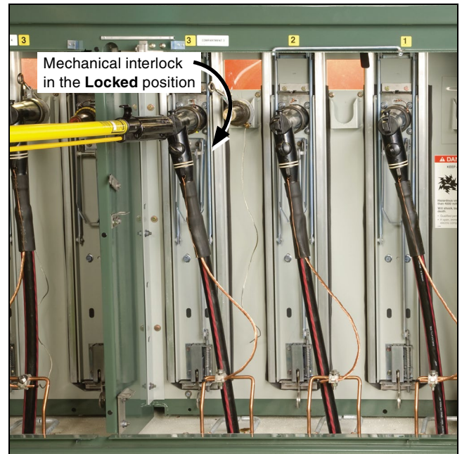
Figure 15. Removing the loadbreak elbow interrupts any load through the fuse to be removed
