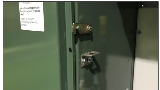
Figure 8. The left-door latching mechanism engaged.
