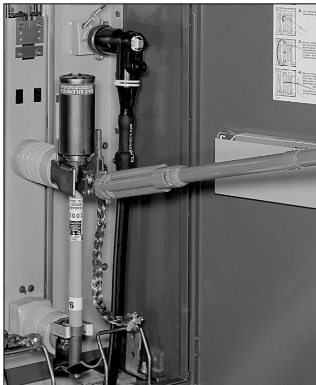
Figure 22. A shotgun stick secured to a fuse pull-ring in preparation for unlatching the fuse.
