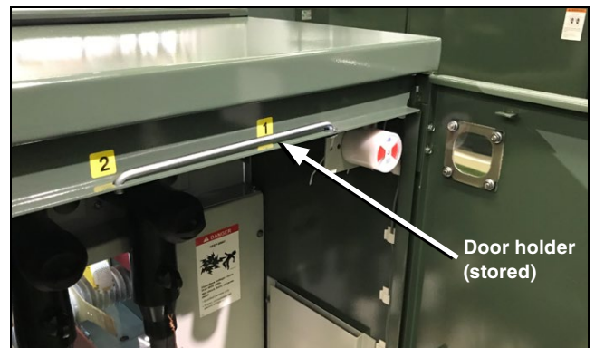
Figure 7. The door holder placed in the storage position to allow the door to close.
