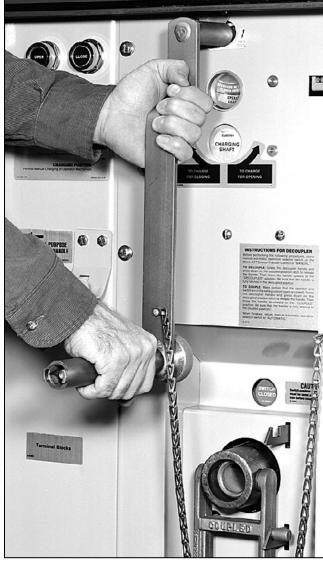
Figure 6. Dual-purpose manual handle inserted in groove of tripping shaft for emergency manual switching if control power is lost and the operator is charged.
