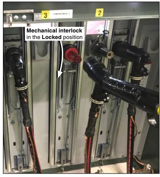
Figure 9. Removing the loadbreak elbow interrupts any load through the fuse to be removed.
