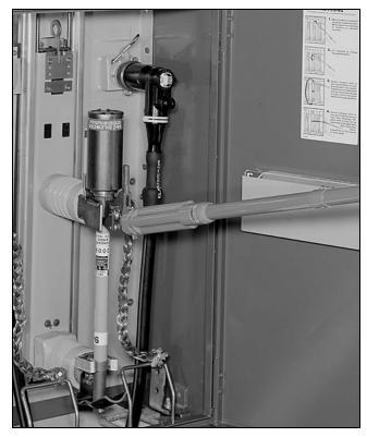
Figure 16. A shotgun stick secured to a fuse pull-ring in preparation for unlatching the fuse.
