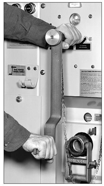
Figure 7. Dual-purpose manual handle on the charging shaft.
