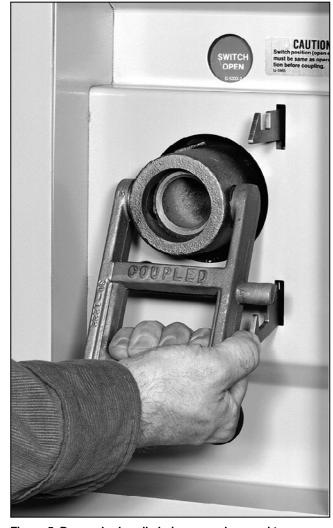
Figure 5. Decoupler handle being moved upward to decouple the switch from the associated switch operator.
