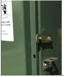
To secure the lefthand door closed, rotate the latch downward over the stop on the outer edge of the door.
