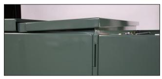
Figure 4. Roof section disengaged from pad-mounted gear enclosure.
