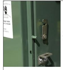
Rotate the latch upward to disengage the left-hand door.
