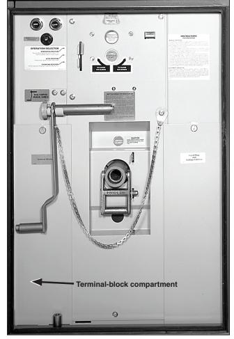
Figure 9. Left side of low-voltage control compartment showing location of left terminal-block compartment—right terminal-block compartment similar—for connection of leads from S&C Current Sensors furnished with optional overcurrent lockout and for customer connections when optional auxiliary switches, remote indication, or supervisory control is furnished. Terminal blocks for options "-Y4" and "-Y6" are in the left terminal-block compartment only.
