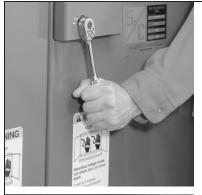
Unlatching Penta-Latch Mechanism with pentahead socket wrench—a distinct click indicates the mechanism is unlatched and recharged.
