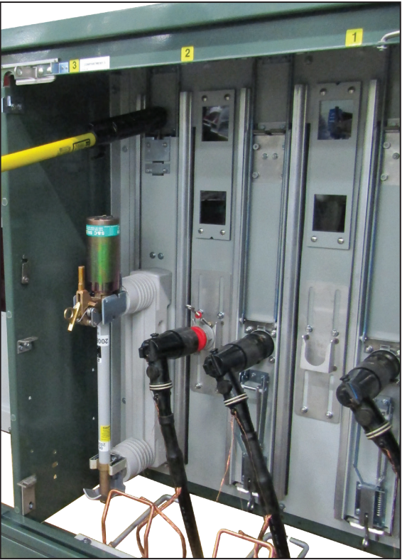
Figure 7. Latching (or unlatching) a TransFuser Mounting in the Open position.
