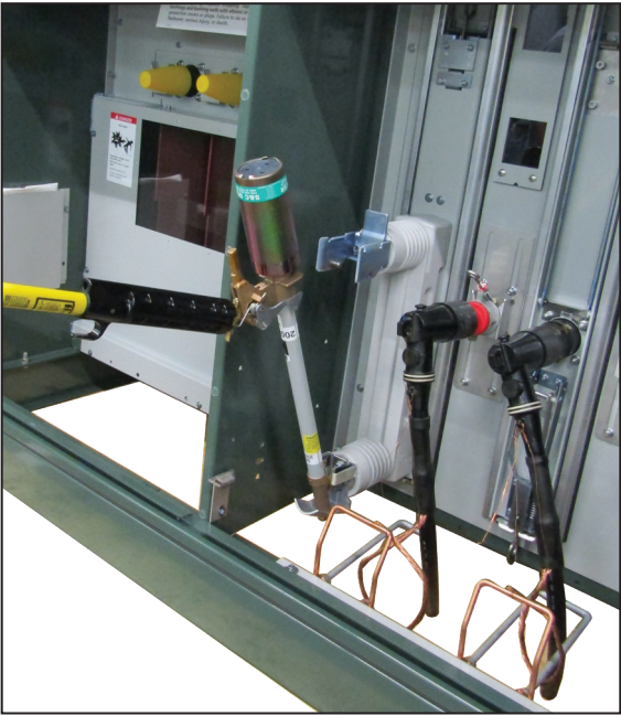
Figure 6. A fuse lowered into the cradle in preparation for latching into a TransFuser Mounting.
