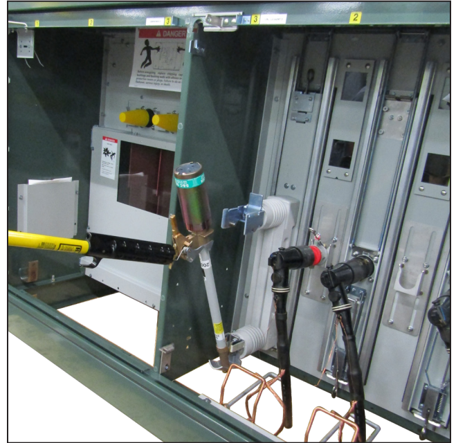
Figure 18. A fuse lowered into the cradle in preparation for latching to a TransFuser Mounting.
