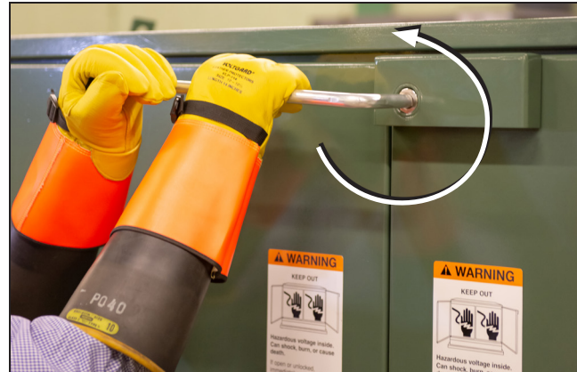
Figure 2. To unlock the doors, turn the pentahead socket wrench 60° counterclockwise against spring resistance until a “click” is heard and the wrench reaches its stop.
