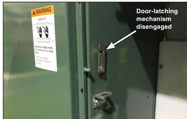
Figure 3. The left-door latching mechanism disengaged.
