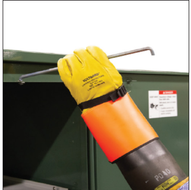
Figure 5. Lift the door holder to allow the door to swing closed.
