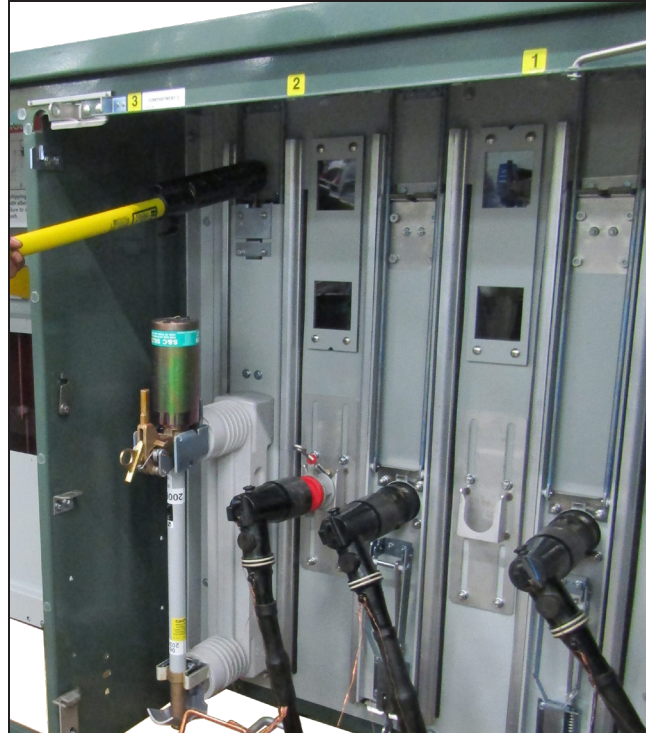
Figure 20. Latching (or unlatching) a TransFuser Mounting in the Open position.
