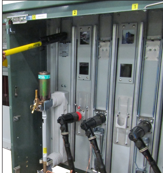
Figure 17. Latching (or unlatching) a TransFuser Mounting in the Open position.
