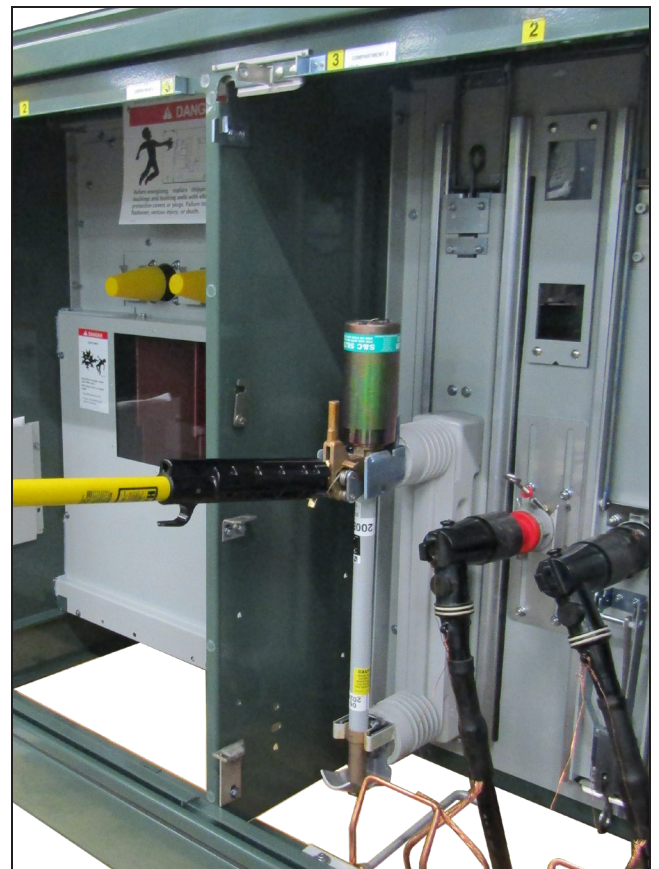
Figure 19. Pull on the fuse assembly by locating the ring of the stick in the opening below the pull-ring.
