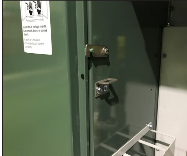
Figure 7. The left-door latching mechanism engaged.
