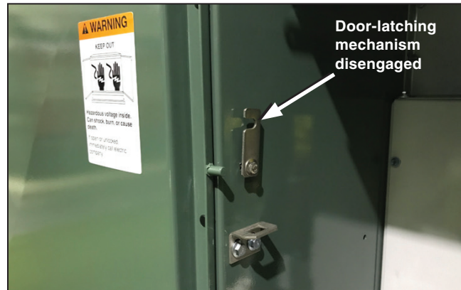
Figure 3. The left-door latching mechanism disengaged.
