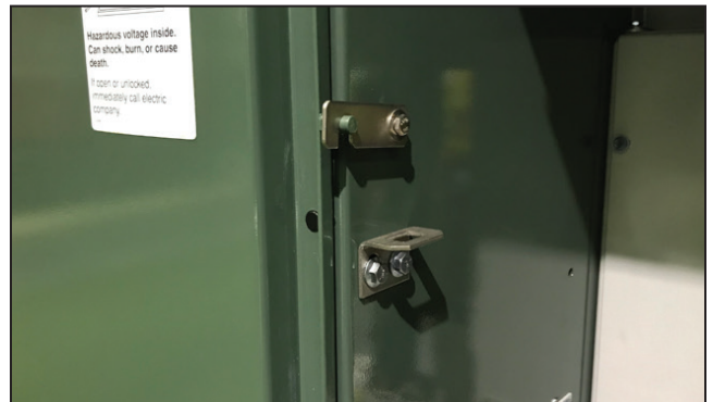
Figure 7. The left-door latching mechanism engaged.
