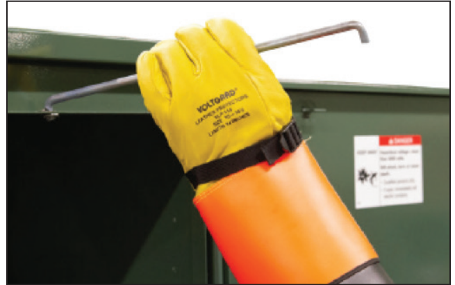
Figure 5. Lift the door holder to allow the door to swing closed.
