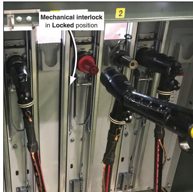
Figure 14. Removing the loadbreak elbow interrupts any load through the fuse to be removed.
