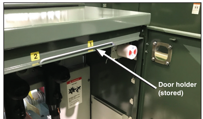
Figure 6. The door holder placed in the storage position to allow the door to close.
