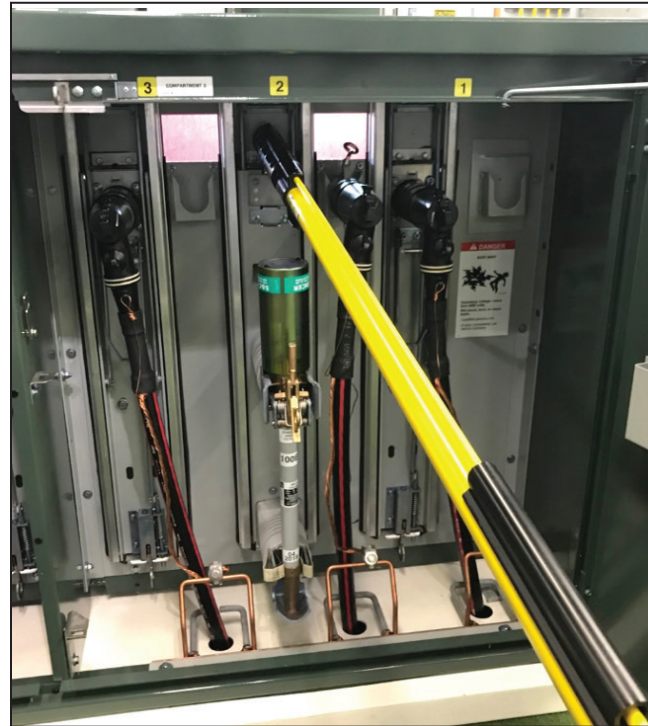
Figure 17. Latching (or unlatching) a TransFuser Mounting in the Open position.
