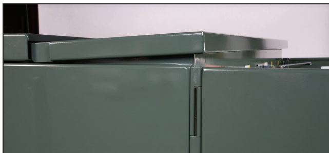
Figure 4. Roof section disengaged from the pad-mounted gear enclosure.
